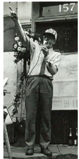
Rev. Calvert at the start of reconstruction work at 157 East 104th Street in 1977.
